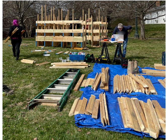
Figure 3. Pavilion assembly in field. The Authors.
