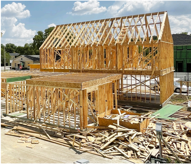
Figure 2. Wood waste on a residential construction site. The Authors.
